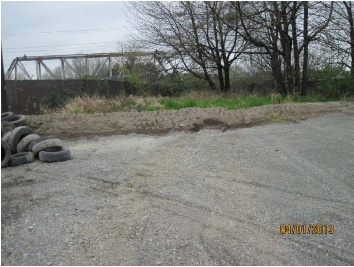
#9 DESCRIPTION: GRADED AND BERMED ALONG THE WESTERN PORTION
